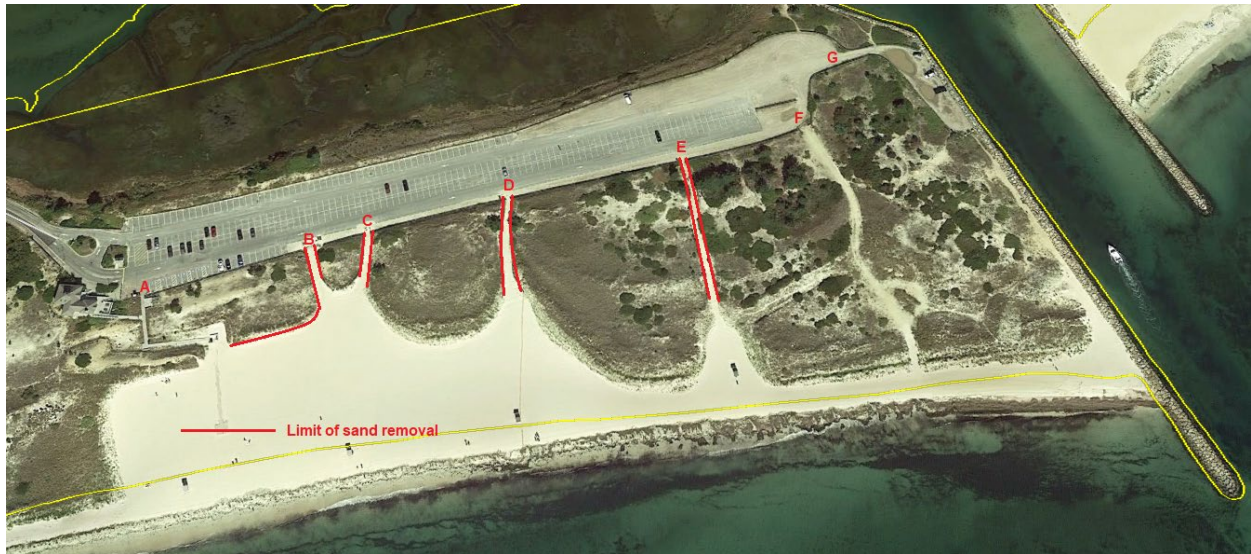
Figure 2. Extent of dune maintenance activities
